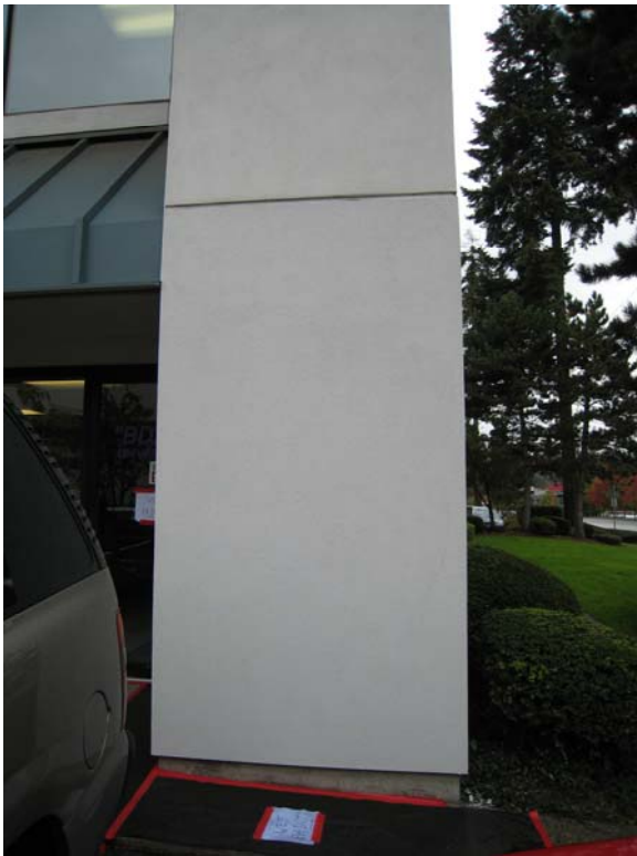
Description: Same as above. Finish coat applied with texture and color matched to existing building color.
