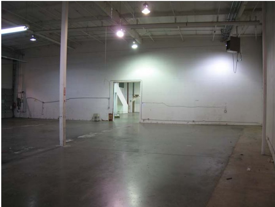
Description: Warehouse demising wall to be demolished.
