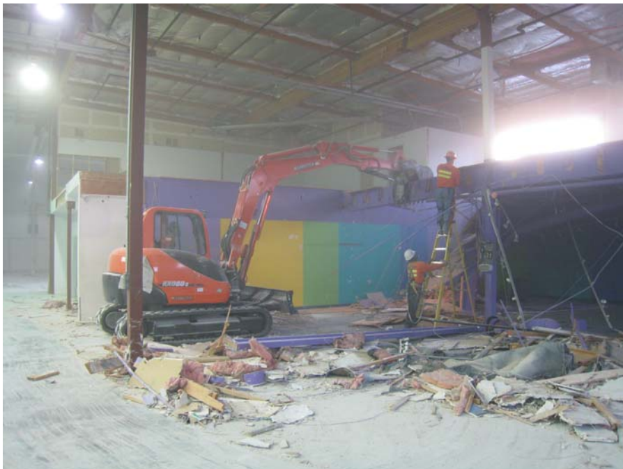
Description: Office Mezzanine glu-lam supports being cut and removed.
