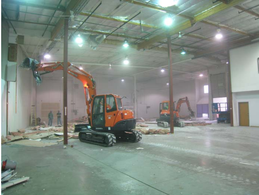
Description: Warehouse demising wall demolition.
