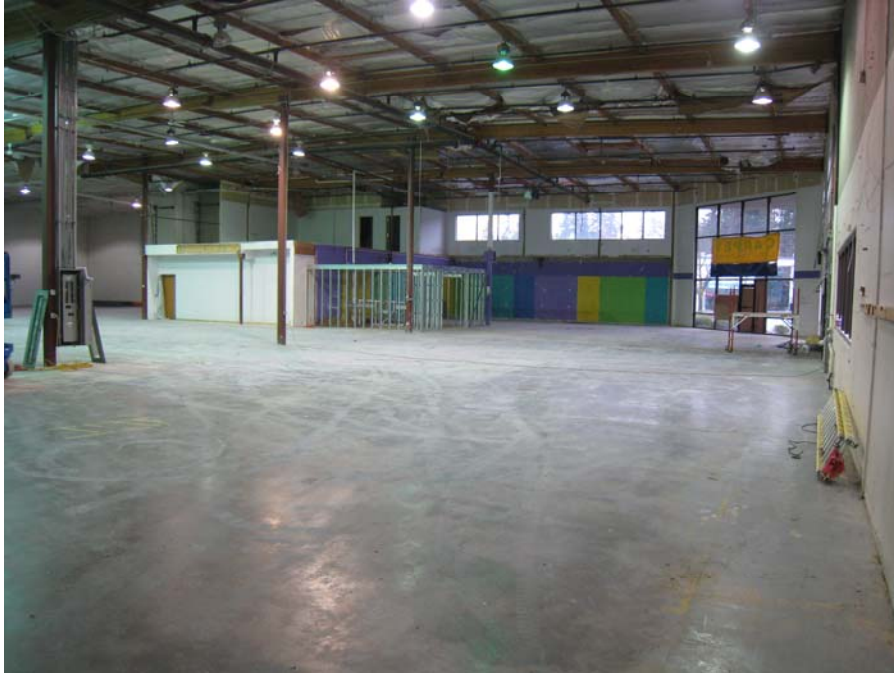
Description: Demolition complete. Framing installed for 2 new restrooms.
