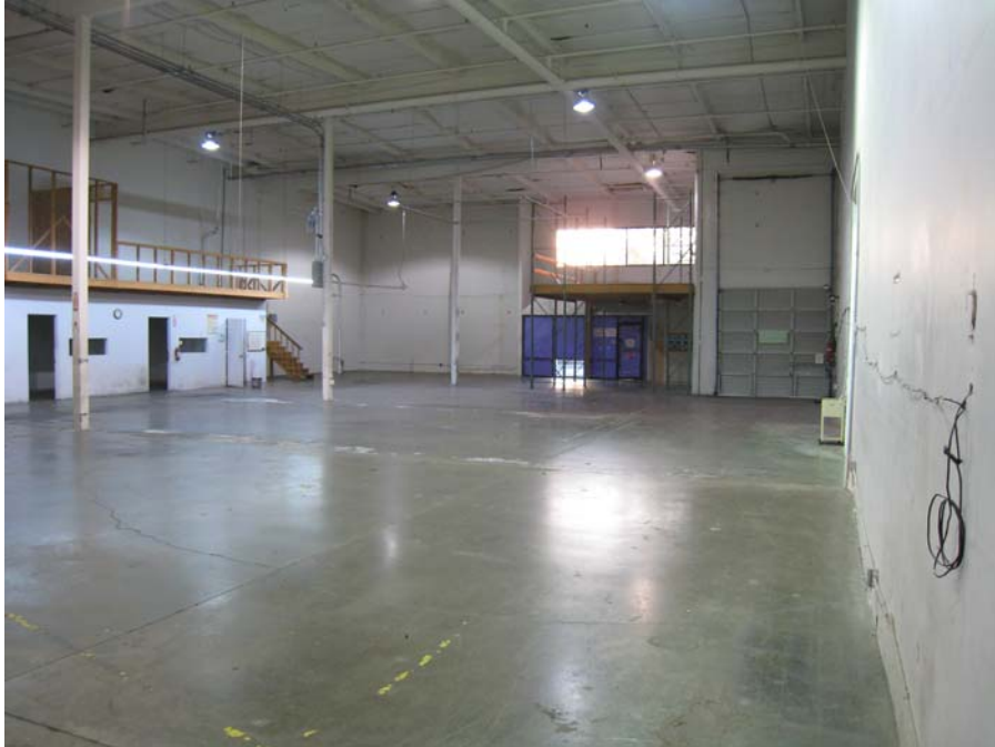
Description: Warehouse office, restroom, metal racking platform to be demolished.
