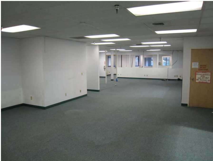
Description: 2 nd Floor Office Mezzanine to be demolished.
