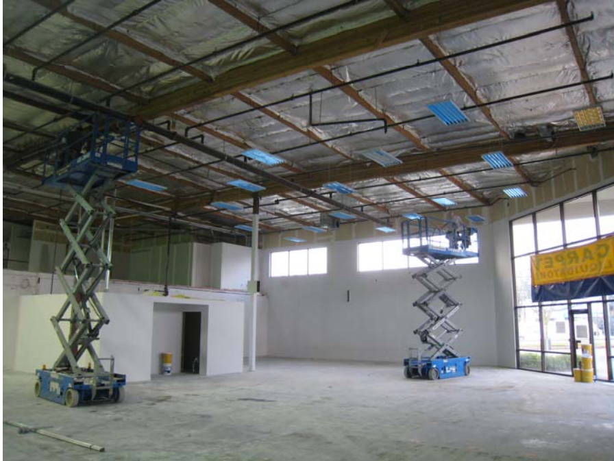
Description: Install new retail area lighting
