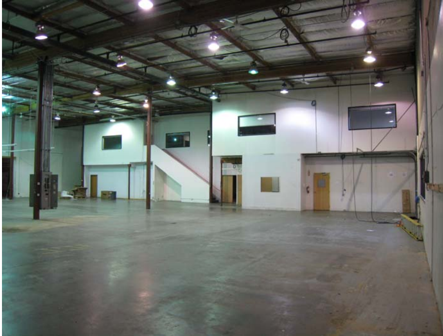
Description: Office mezzanine to be demolished.
