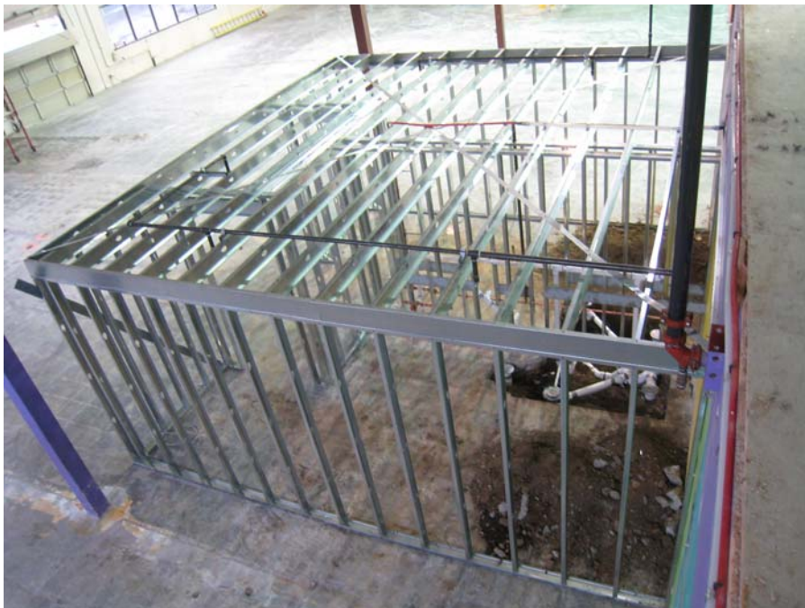
Description: Framing and plumbing rough-in complete after saw-cut warehouse floor.
