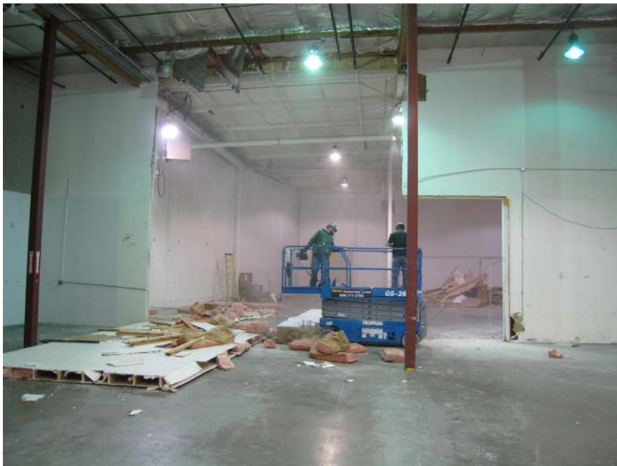
Description: Warehouse Demising wall being demolished.
