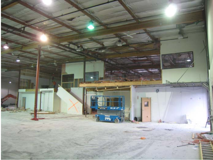
Description: Office Mezzanine being demolished.
