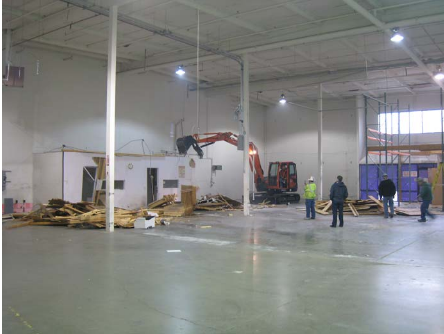
Description: Warehouse office, restroom, metal racking platform being demolished.
