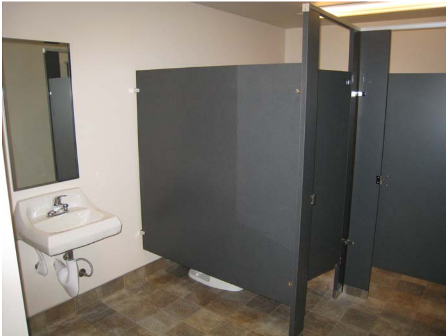
Description: Finished Woman's restrooms with new sink, toilets, partitions etc.
