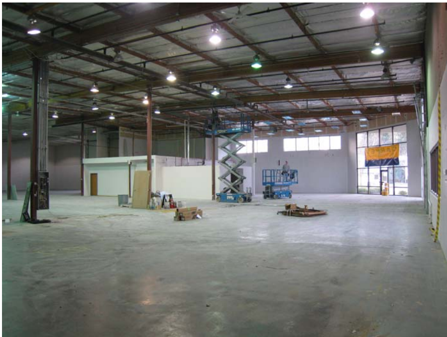
Description: Painting and install of new retail lighting.
