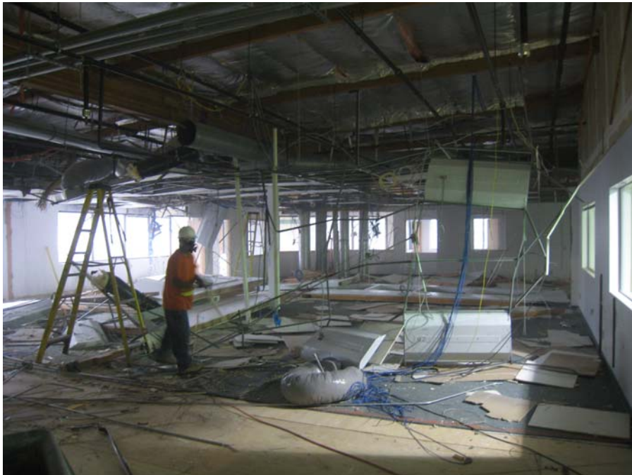
Description: 2 nd Floor Office Mezzanine being demolished.
