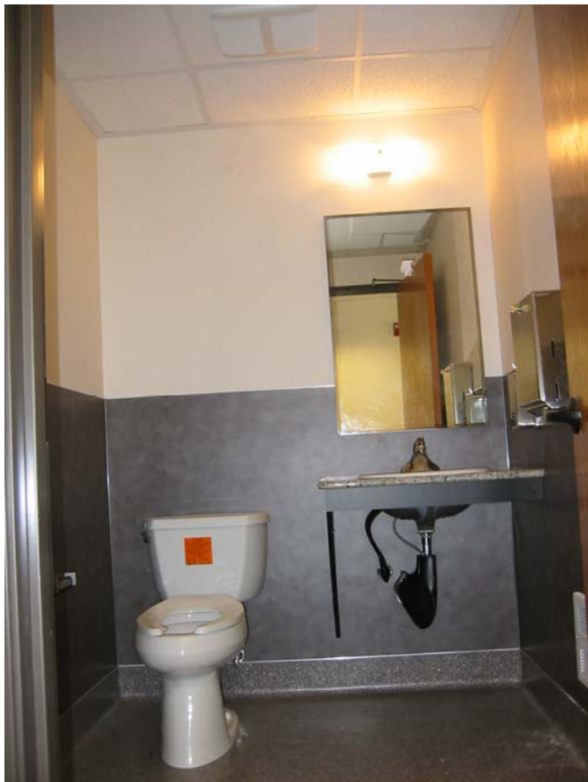
Description: Bathroom #1 ADA. All new fixtures, accessories, ADA grab bars and heater. Sheet vinyl flooring with wainscot. New granite counter and sink.
