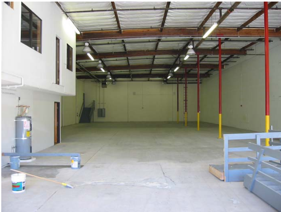
Description: Warehouse Floor. Completed and sealed.
