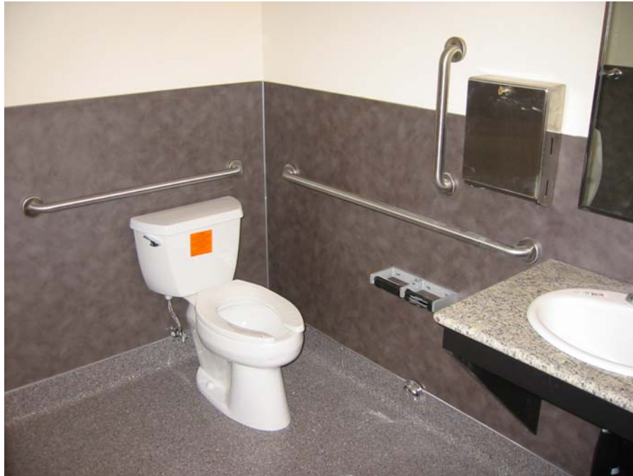
Description: Bathroom #1 ADA. All new fixtures, accessories, ADA grab bars and heater. Sheet vinyl flooring with wainscot. New granite counter and sink.
