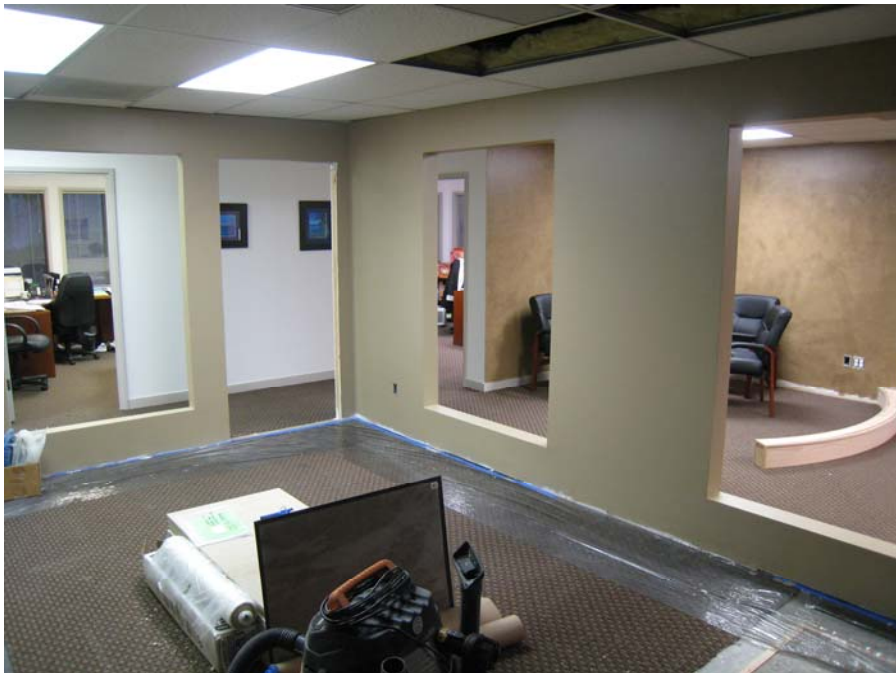
Description: Conference Room rebuilt and ready for doors and glass block.
