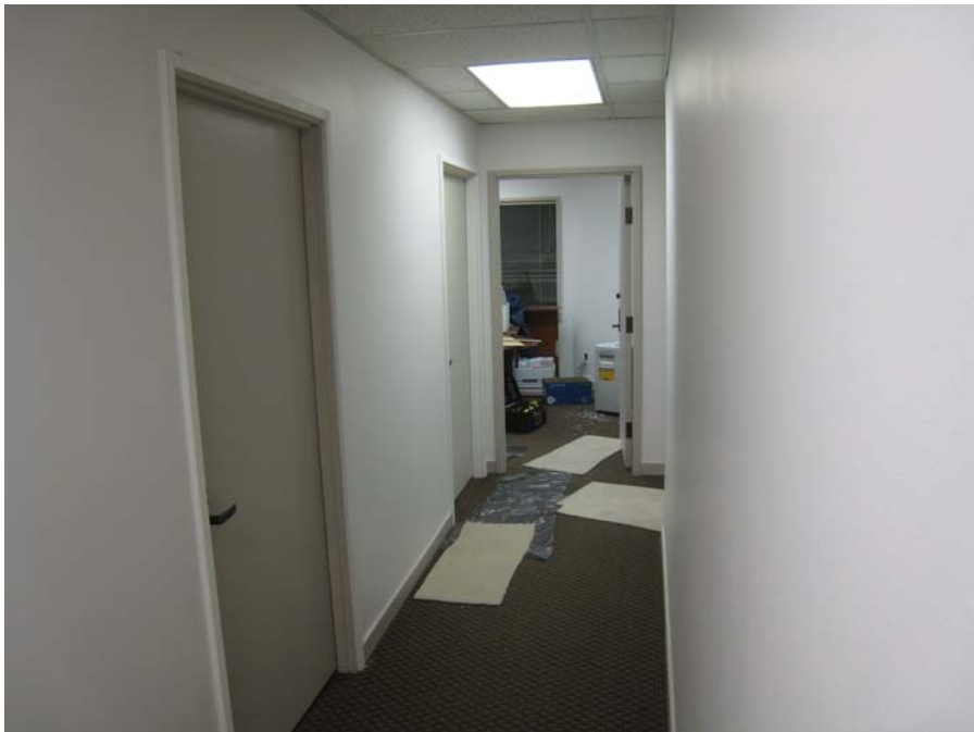
Description: Hallway with new offices completed with new doors and trim.
