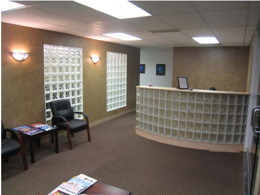
Description: Reception area finished with wall sconces, curved reception desk with glass block and electrical work completed.
