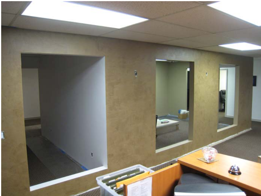
Description: Glass block wall rebuilt and ready for glass block installation.
