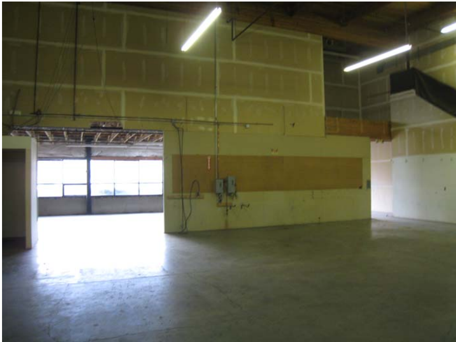
Description: Short warehouse demising wall to be demolished.
