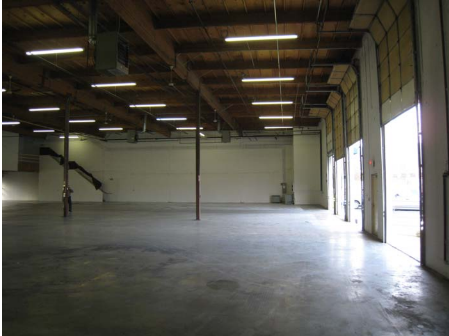
Description: Warehouse complete with re-balanced lighting, removal of power drops and 4" electrical gutter, painted, floor scrubbed.
