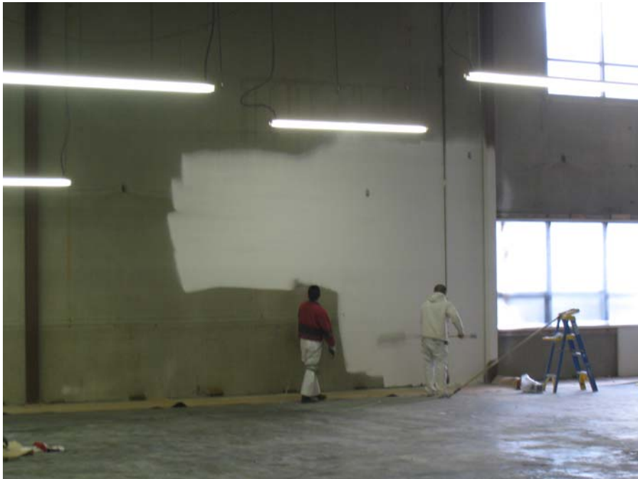
Description: Warehouse painting beginning.
