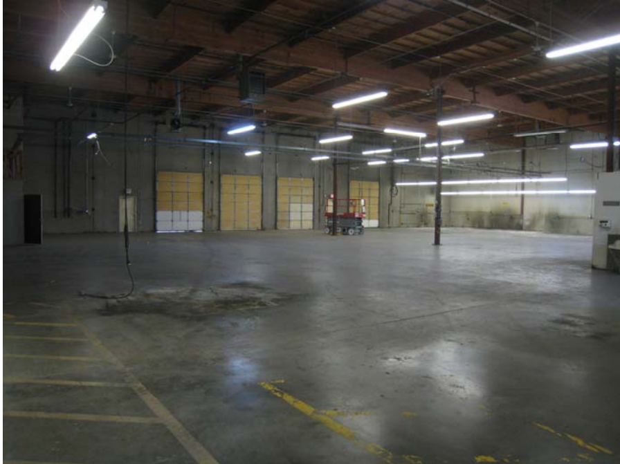
Description: Warehouse existing condition.
