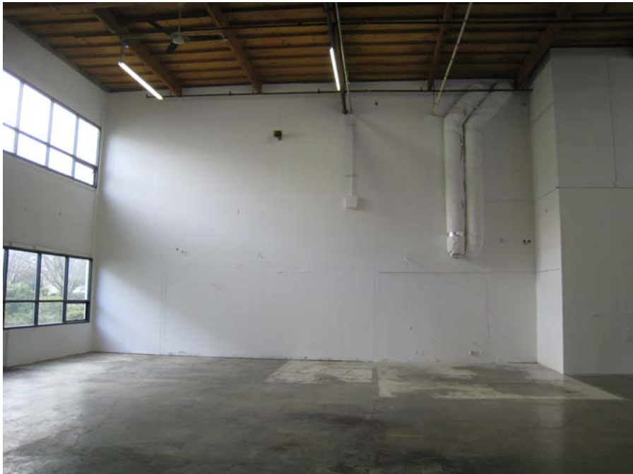
Description: Completed warehouse office area, painted, and cleaned.
