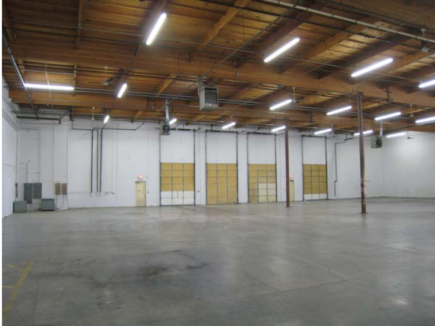
Description: Warehouse lighting re-balancing into “rows”, floor scrubbed, warehouse painted.
