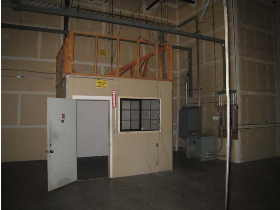
Description: Existing warehouse supervisor's office to be removed.
