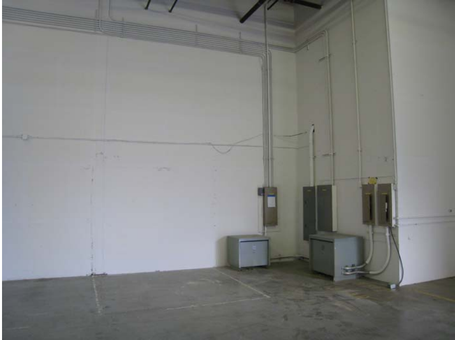
Description: Warehouse supervisor's office demolished, electrical area cleaned up and painted.
