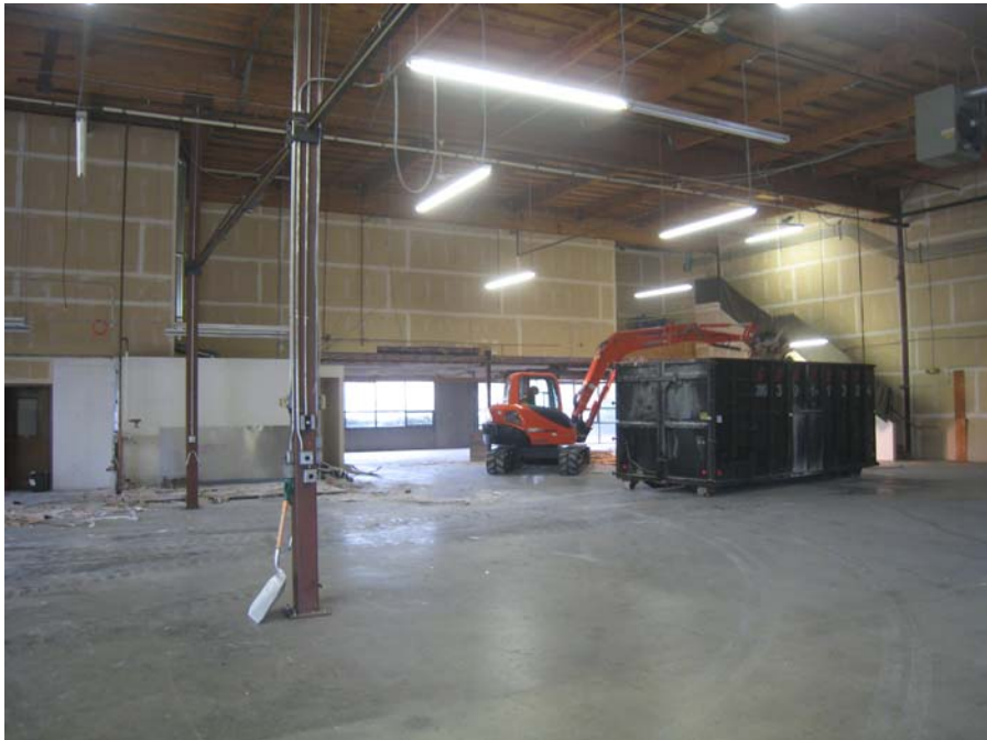
Description: Start of demolition of warehouse demising wall.
