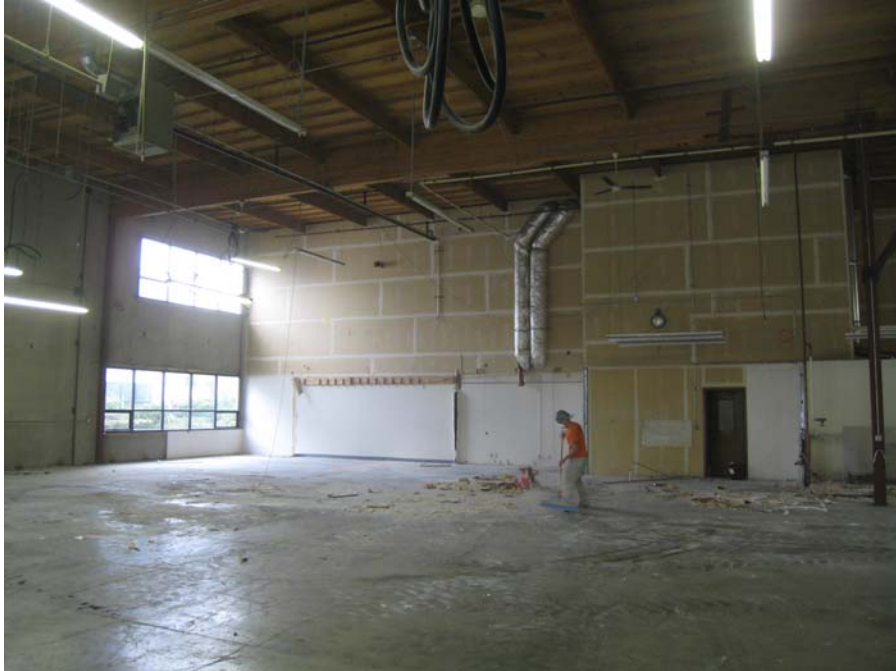
Description: Warehouse office demolished.
