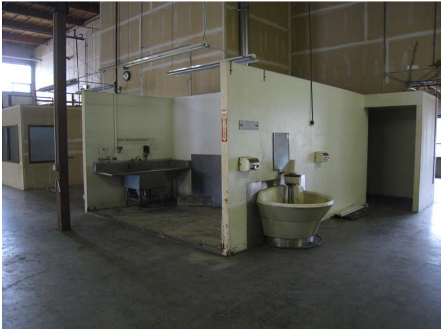
Description: Existing wash-down area with sinks to be removed.
